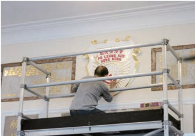
▲ 修復人員為關帝廳內的局徽及碑石上色及重貼金箔。 Conservation specialist repainted the Kuk's emblem and gilded inscriptions with gold leaves in the Kwan Ti Hall.
