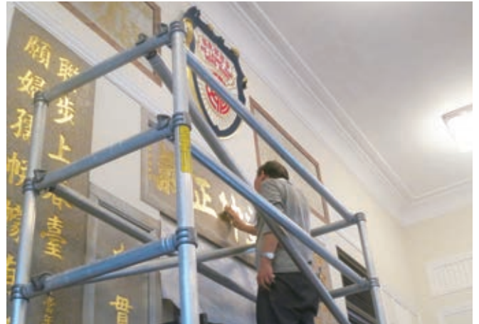
▲ 修復人員為關帝廳內的局徽及碑石上色及重貼金箔。 Conservation specialist repainted the Kuk's emblem and gilded inscriptions with gold leaves in the Kwan Ti Hall.
